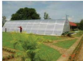
Figure 4. PV-ventilated greenhouse dryer (Janjai et al., 2009).
